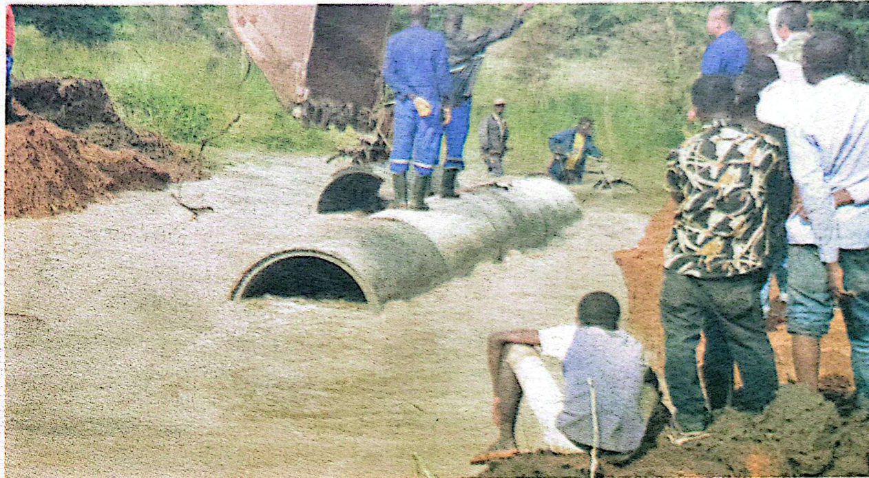
Efforts. Culverts are installed at Lorengchora Bridge in Napak District following the floods on Tuesday. PHOTO BY STEVEN ARIONG
